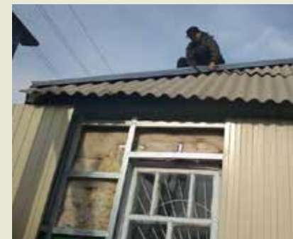
Repairing the House of Prayer.
