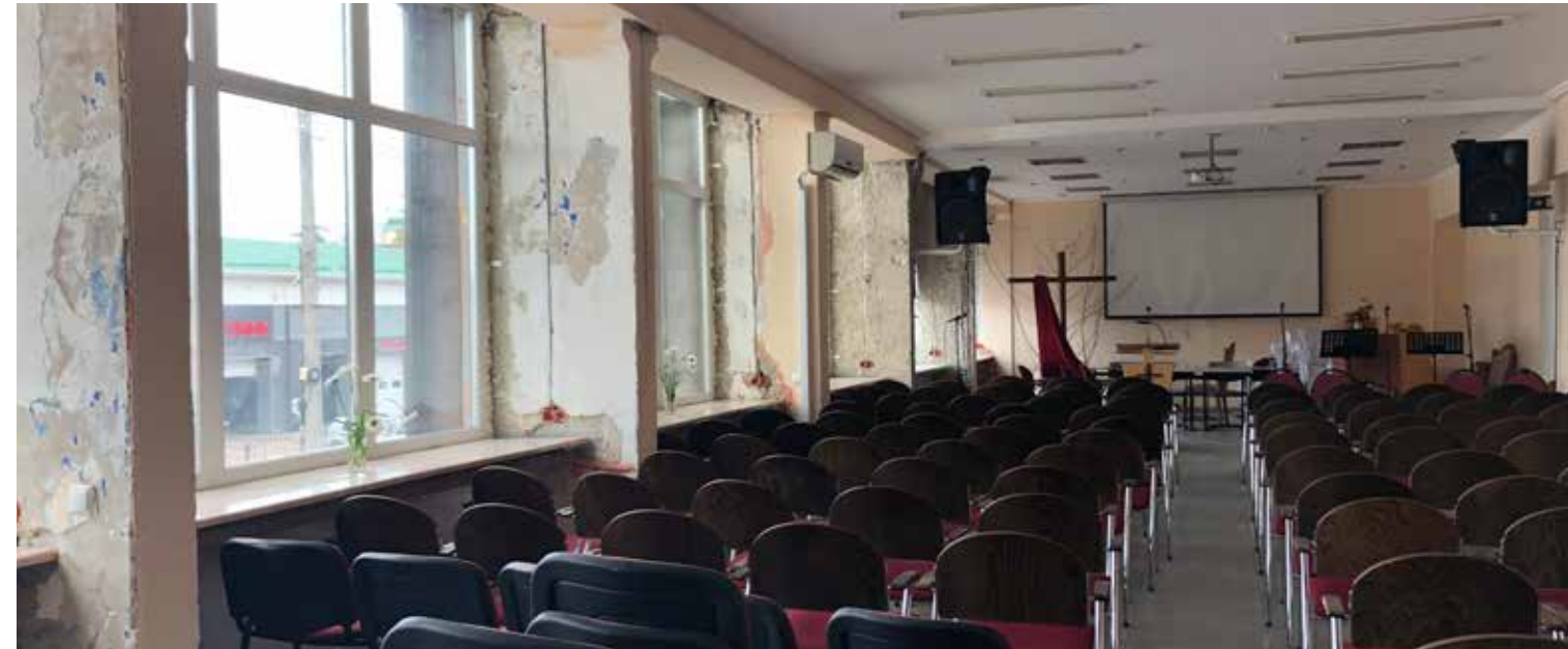
The Second Baptist church was damaged by three shells.
