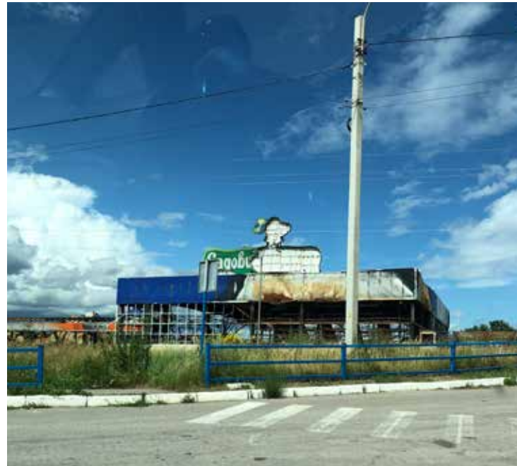
Many homes and businesses are not repairable.
