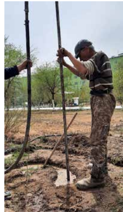
Drilling the well.
